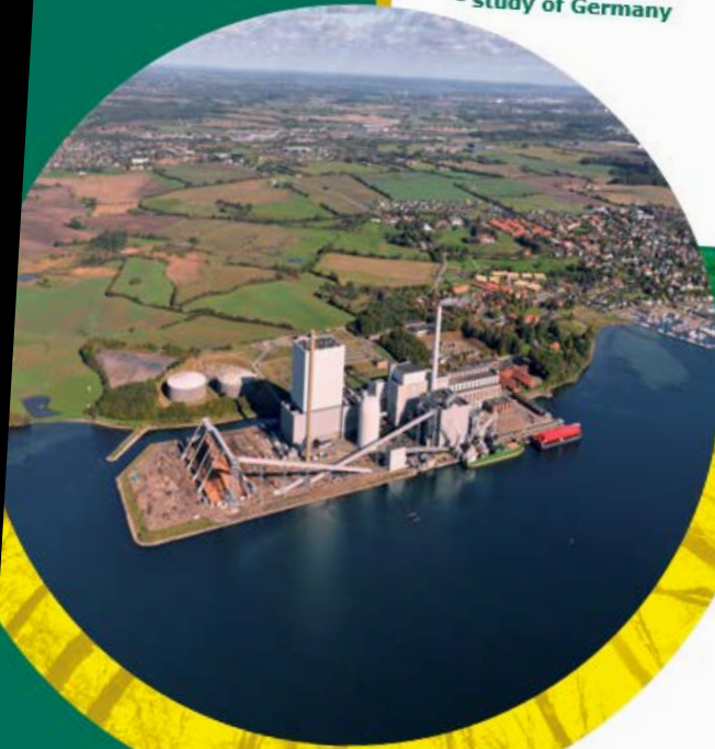
Skarboek CHP plant, Denmark. Photo: Ørsted
